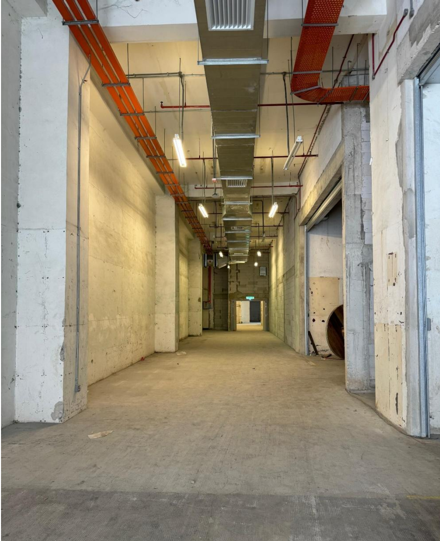
Common Walkway Access to Loading Bay & Cargo Lift
